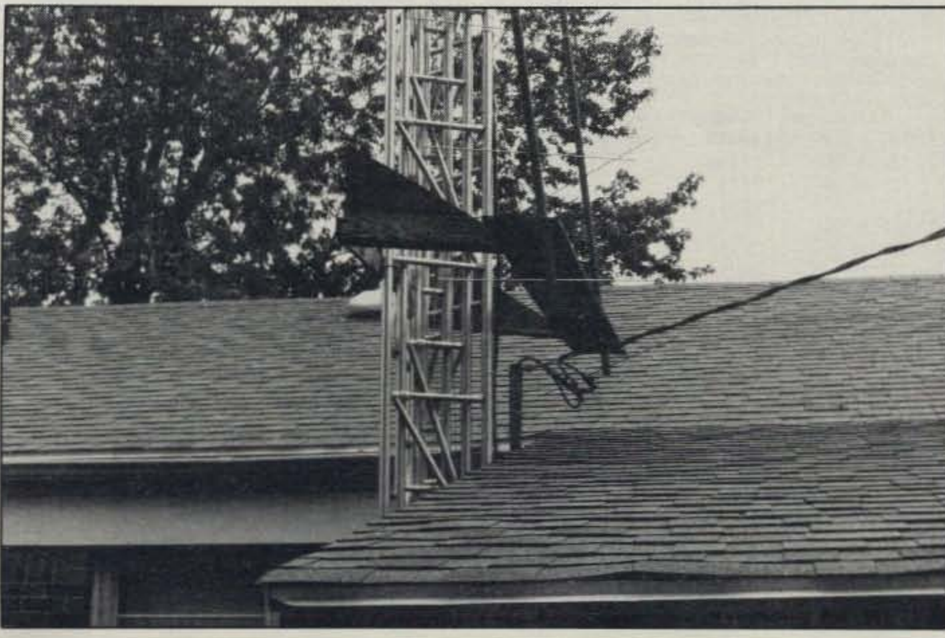
Fig. 4—A simple wooden cradle steadies the antenna during high winds—and also out of the power-line feed.
