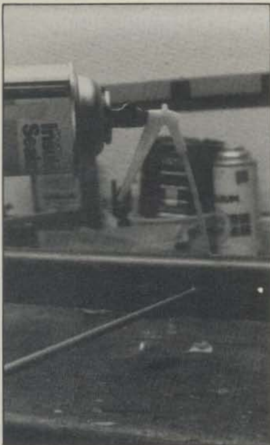
Fig. 8—A final squirt of foam insulation. It also made the boom 100% draft free.
